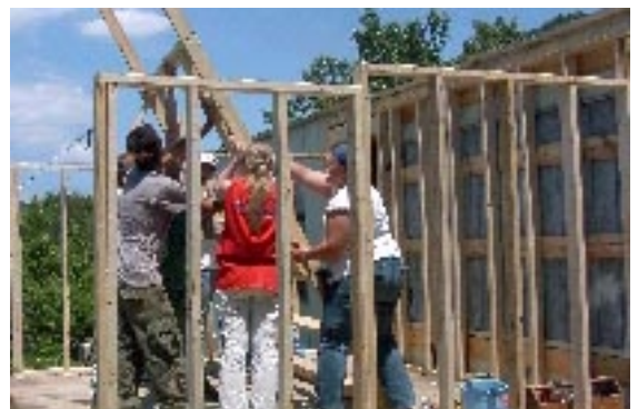
The walls for a new bedroom go up at ASP.
