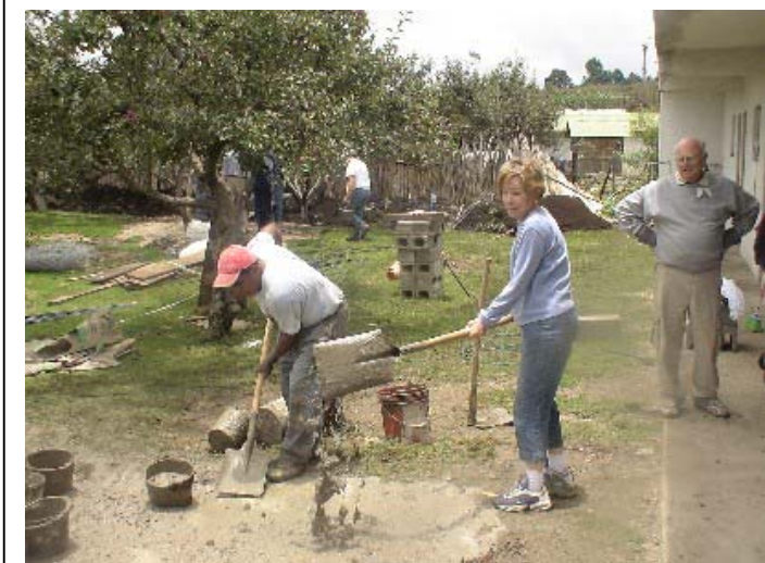
Elizabeth Gross helps mix cement. (Tom Purcell is on the right.)
