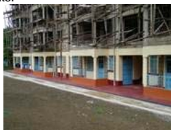
The 4 story flats with 4 apartments completed for interns
