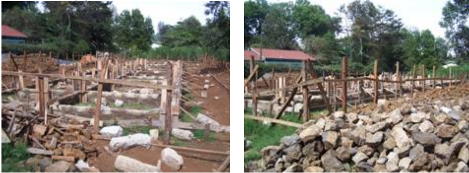
The foundation work at our future 4 story staff flats
